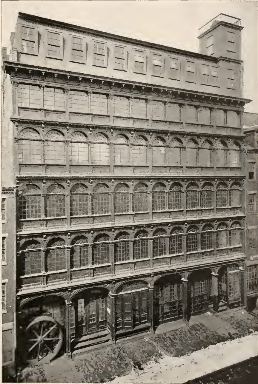
IRON BUILDING—G. T. McLAUTHLIN & CO.
